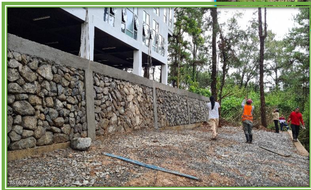
Slope Protection at the JHMC Office Complex,
