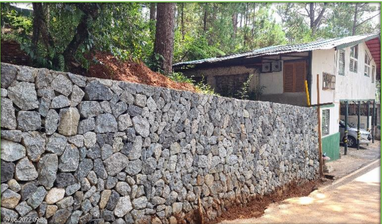
Slope Protection at the JHMC Office Complex,
