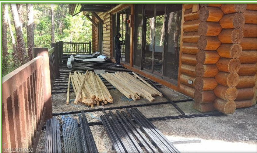
Laying-out and installation of WPC flooring.
