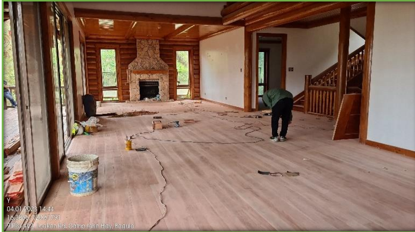
Removal of existing flooring, installation of Tongue and Groove (T & G) flooring.
