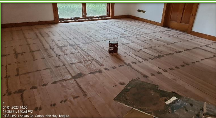
Removal laying-out and installation of T & G flooring.
