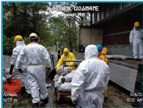
Actual weighing and loading to truck on August 6, 2021. SSD and EAMD – EMD Personnel were there monitoring the activity
