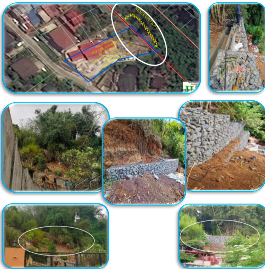
Slope Protection at Hillside Barangay
