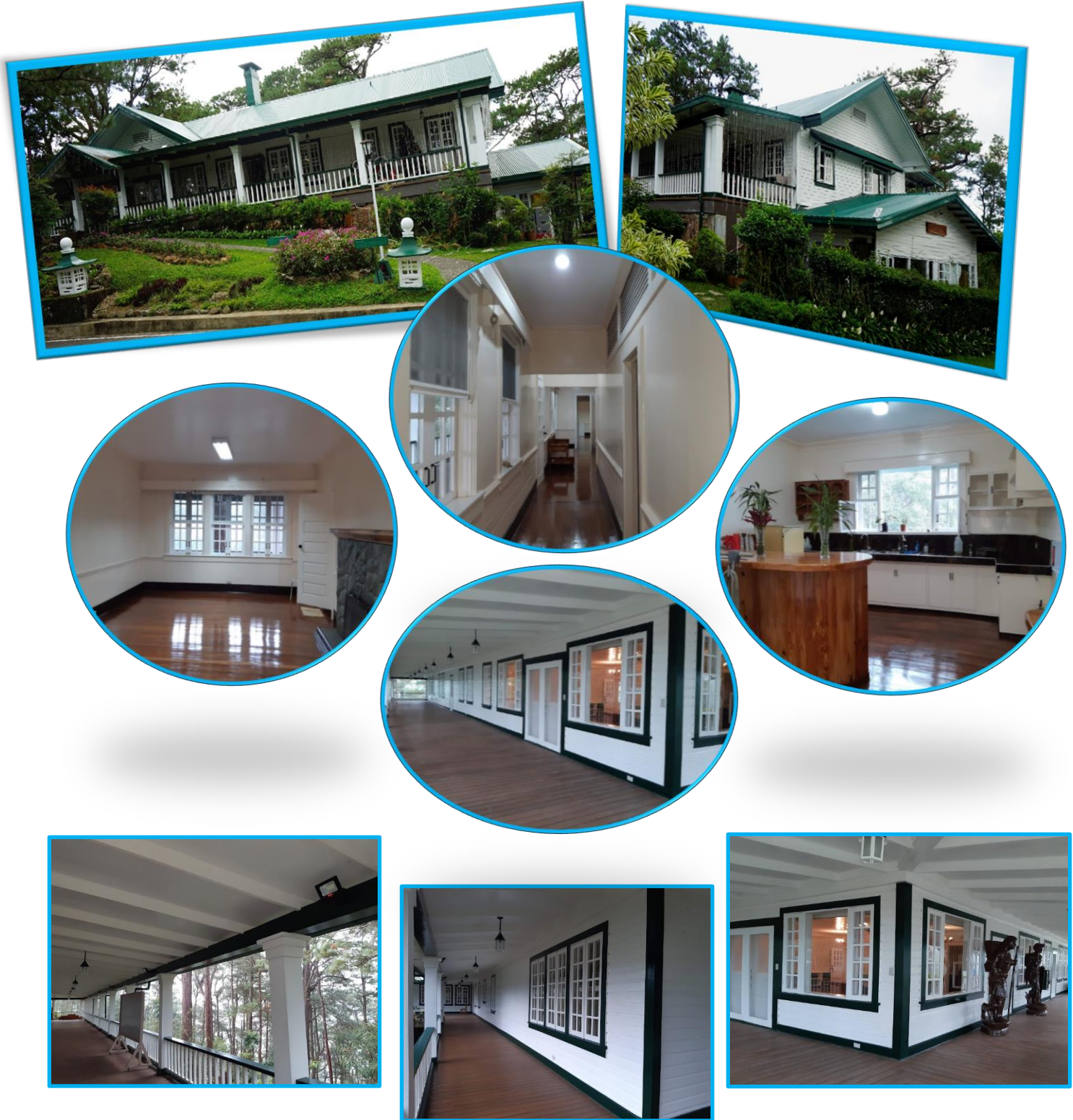
Rehabilitation of Bell House Phase 3
