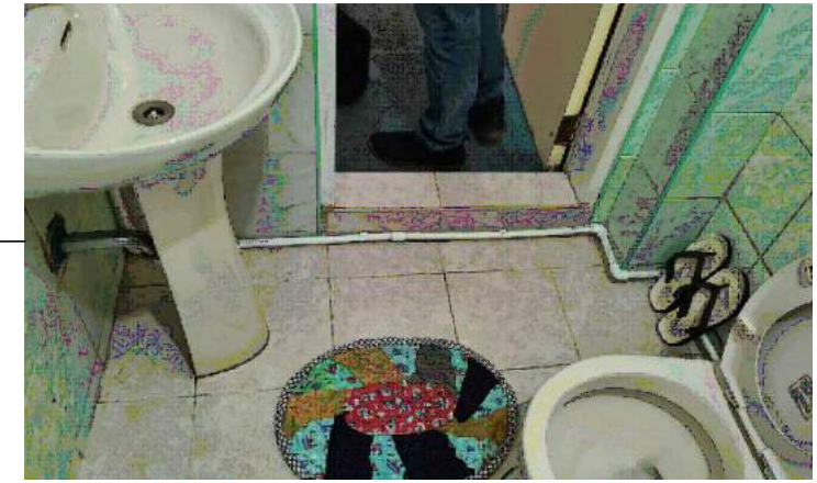
- EMBEDMENT OF EXPOSED PIPING SYSTEM - INSTALLATION OF CERAMIC TILES
