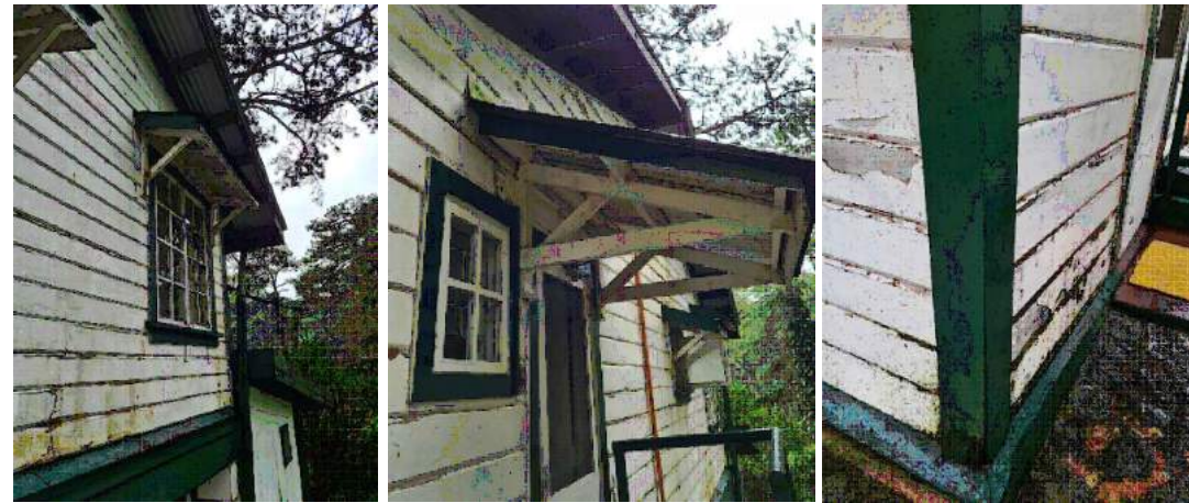
- REPAINTING OF EXTERIOR WALLS - REPLACEMENT OF WOODEN WINDOWS TO ALUMINUM CASEMENT - REMOVAL AND REPLACEMENT OF WINDOW EAVES
