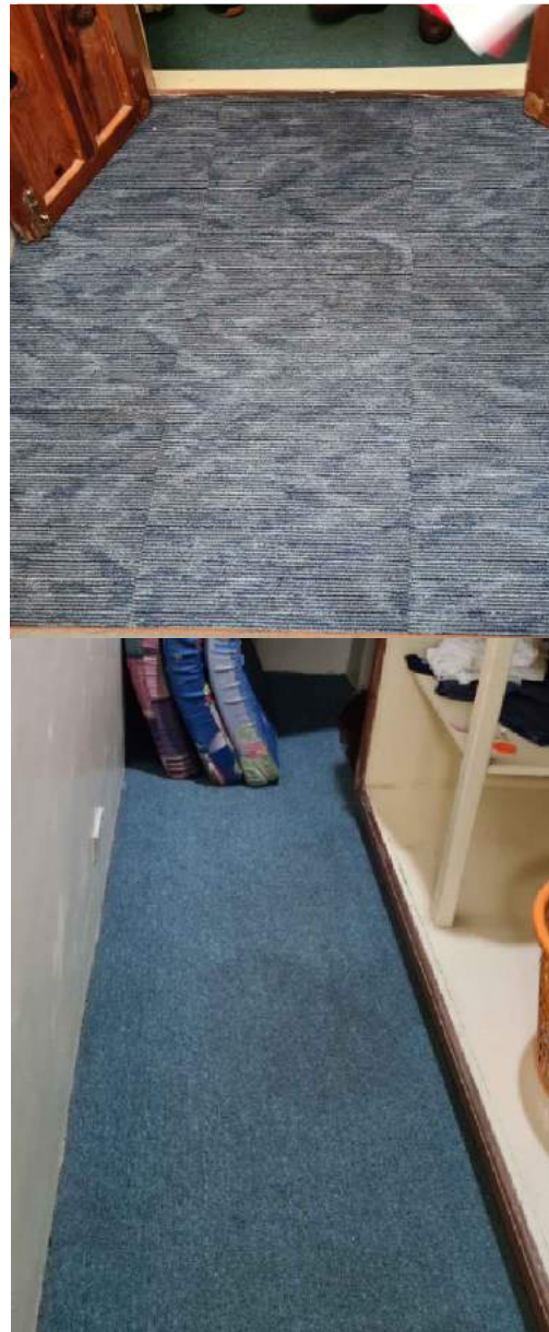
- REMOVAL OF CARPET AND REPLACEMENT OF CERAMIC TILES
