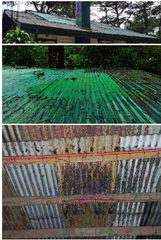
- REMOVAL AND REPLACEMENT OF EXISTING GI ROOF SHEETS, GUTTER, INSTALLATION OF ROOF DRAINS W/ STRAINER
