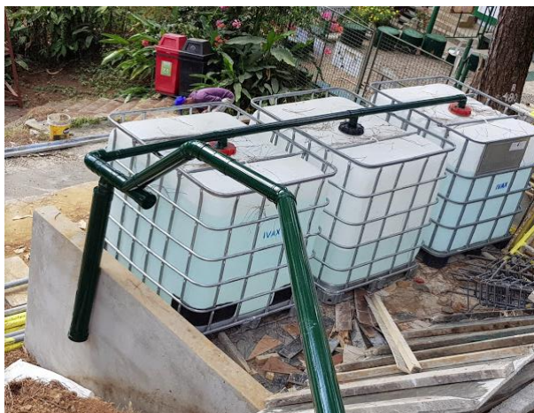
The newly-installed rainwater harvesting facility at the Historical Core.
