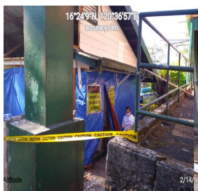
i-Advance Philippines conducting a continuous asbestos ambient air sampling before and during the dismantling and demolition activities.
