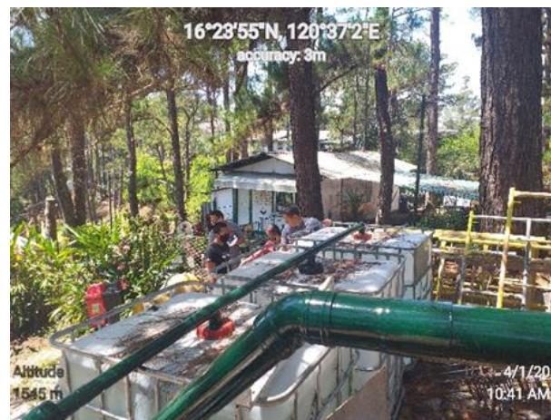
The newly-installed rainwater harvesting facility at the Historical Core.
