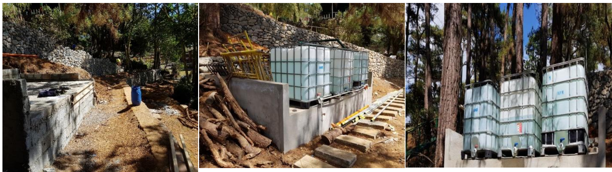
The installed rainwater harvesting tanks has concrete pedestal.
