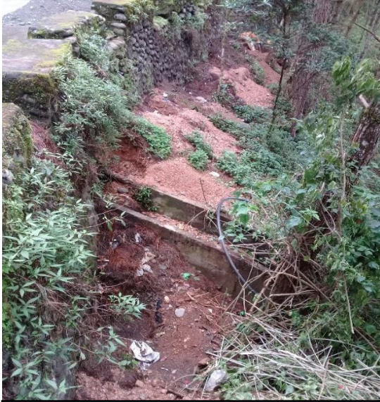
Photos of the Before the Installation at the MOOG-PEZA Fence
