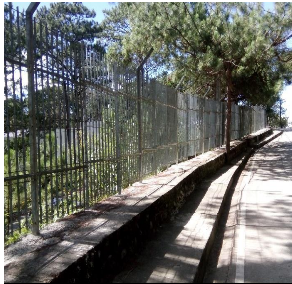
Photos of the After the Installation at the MOOG-PEZA Fence
