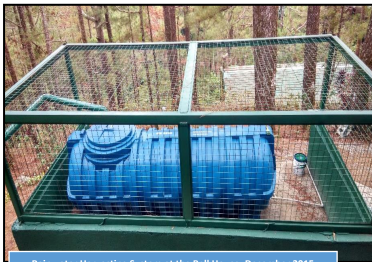
Rainwater Harvesting System at the Bell House, December 2015
