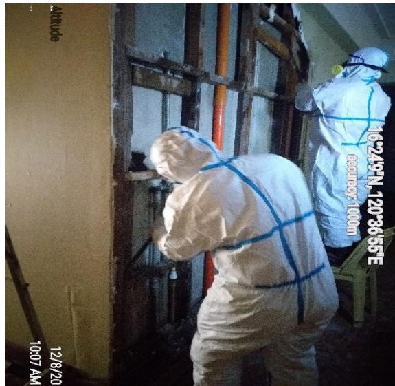
Left: Chemical handling Safety Orientation and Meeting with JHMC personnel following confirmation that there are asbestos materials at the Igorot Lodge toilets' walls and ceiling. Right: Initial dismantling of some asbestos at Igorot Lodge.
