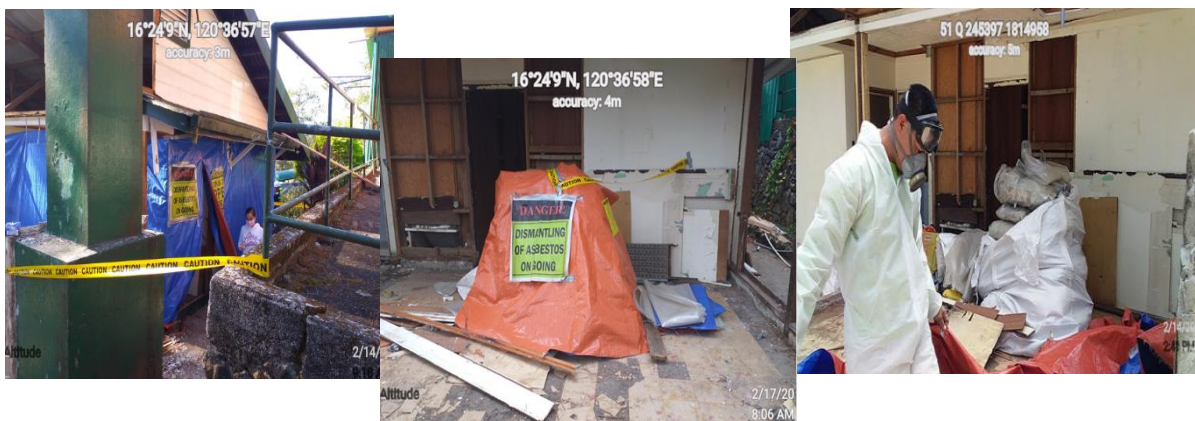
Inspection of final layout of H- Frame scaffolds, air monitoring device, PE liners and signage prior to commencement of demolition works.
