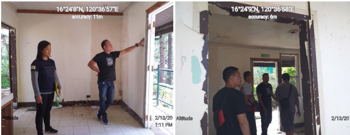
Dismantling Works of Asbestos Materials following DAO 2000 – 02 / Chemical Control Order for Asbestos: Safety and Work Methodology Review, toolbox meeting, and final assessment prior to commencing main works.
