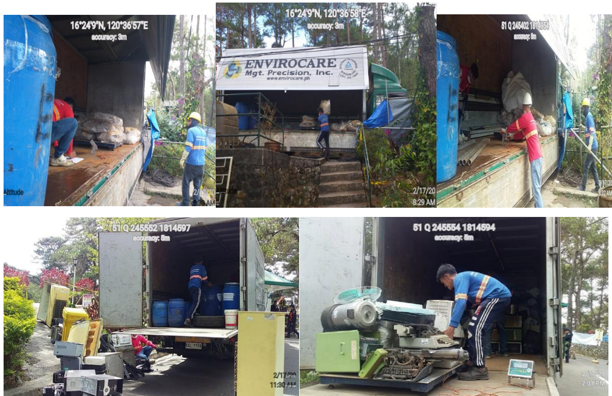
Hauling out and loading into truck/ vehicle covered by the Permit to Transport from EMB- Region III going to Metro Clark Waste Management Facility in Capas, Tarlac. (February 17, 2020)
