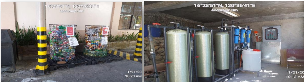
EAMD-Environment Management Division checks on Environment Compliance of locators: photo of the Solid Waste Management and STP control center of IHG.
