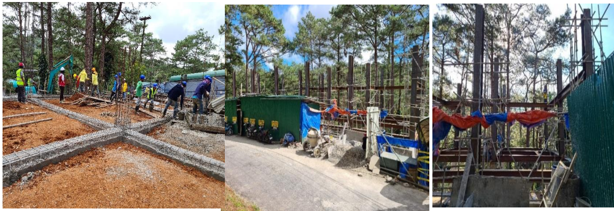
Photos taken during the ongoing rehabilitation works.
