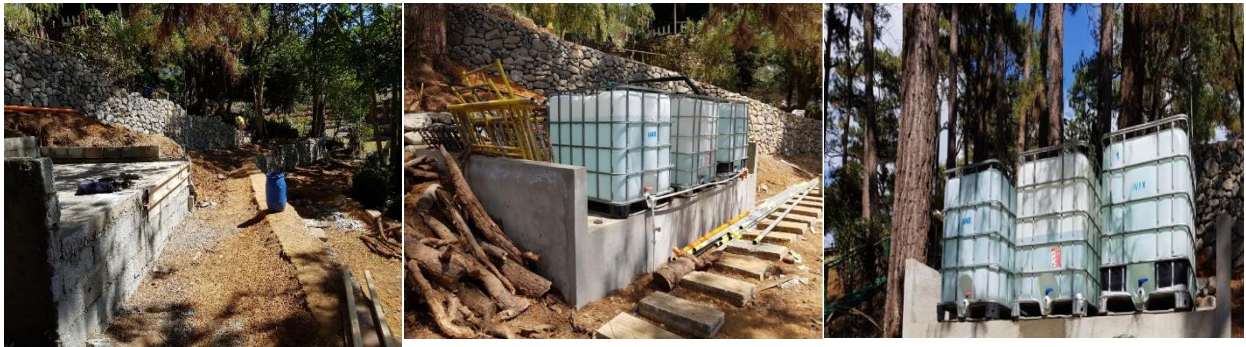
The installed rainwater harvesting tanks has concrete pedestal.
