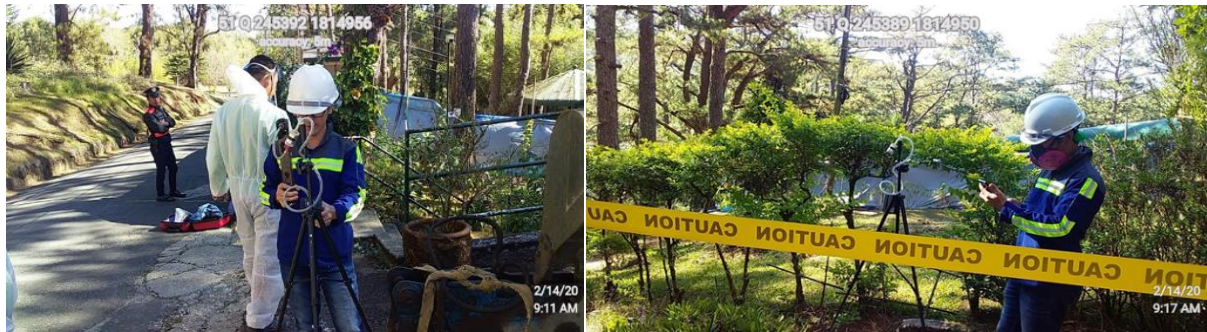
i-Advance Philippines conducting a continuous asbestos ambient air sampling before and during the dismantling and demolition activities.
