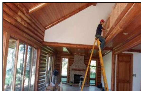
Rehabilitation of VOA Loghome Unit Nos. 3 and 5 (on-going implementation)
