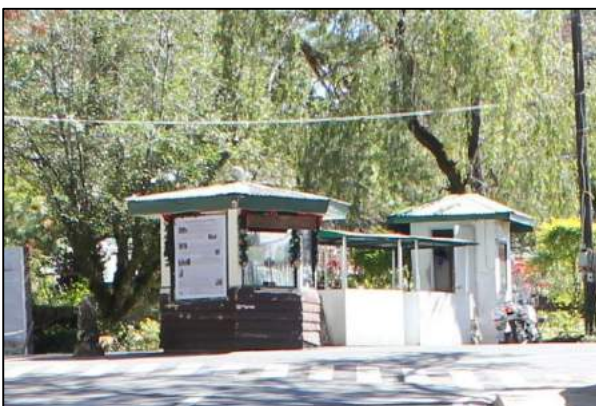
Photo of the area before the repair
