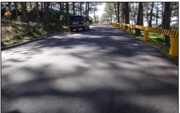
Photo of the area after the repair
