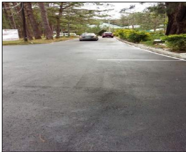
Photo of the area after the repair
