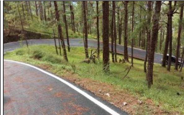
Photo of the area after the repair
