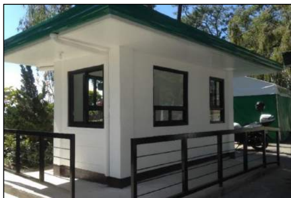
Photo of the area after the repair
