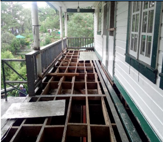
Photos of the Before Rehabilitation of Bell House Porch Flooring and Ceiling
