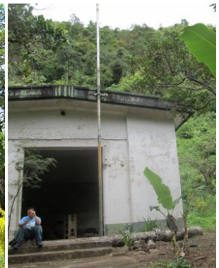
Mini-Hydro Power Plant
