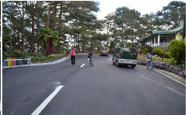
Bell House Driveway
